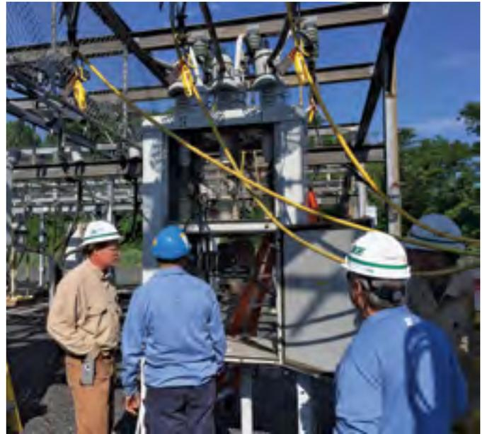
CBS Northeast tested a 15-kV, 1200-A vintage Westinghouse vacuum breaker that the utility thought might have a questionable vacuum interrupter.
